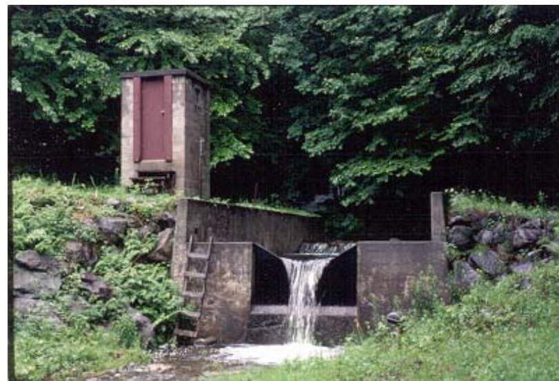
Weirs built on streams to measure volume of water leaving each small watershed ( outputs )
